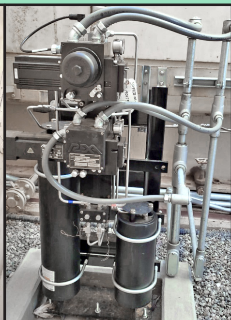
Remote-Mounted Power Module and Accumulator
