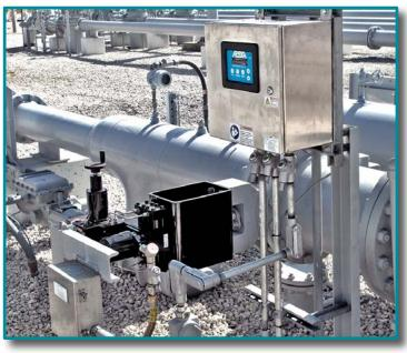
control interacts from one pump station to another, meaning pressure fluctuations at one station will affect all other pump stations on the pipeline. Our actuators provide fast response to pressure disturbances including starts, stops and throttling flow rate changes. They also provide **fast response** to setpoint adjustments at one station in order to achieve the desired flow rate and pressure at another.
