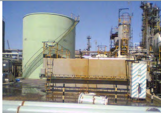
Basin in petrochemical complex
