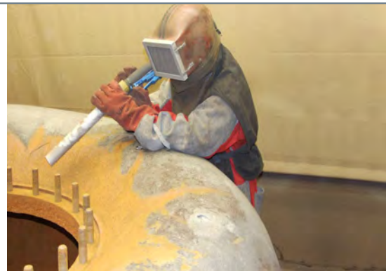
Thorough surface preparation.
