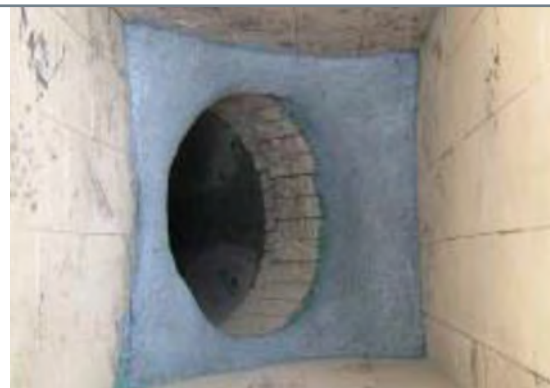
Installation of ARC BX5 .
