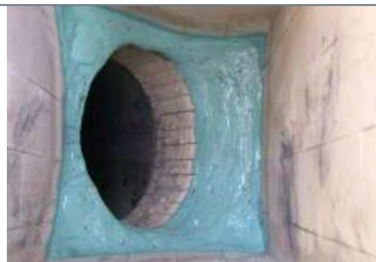
ARC BX5 with ARC S2 topcoat cures rapidly, allowing fast return to service of chute.
